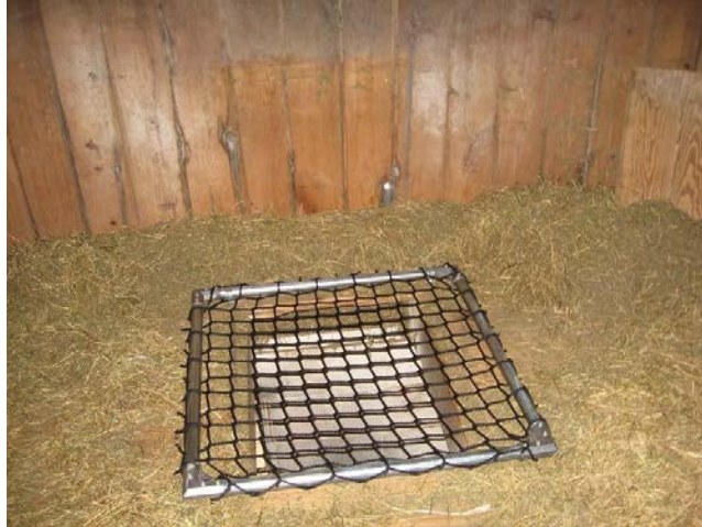
Figure 1: Hay hole cover preventing falls and allowing hay loft ventilation.
